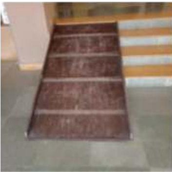
Divyangan Friendly Ramp
