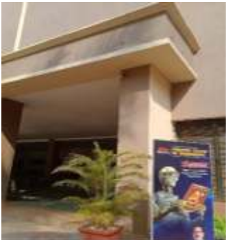
CCTV Camera [Entrance]
